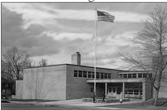
West Annapolis School, 1955 structure
