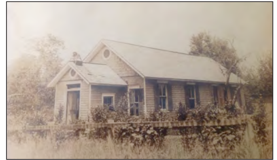
Two-room schoolhouse, 1910 structure
