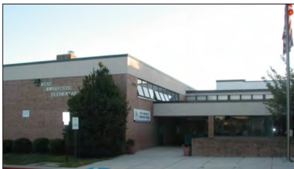
West Annapolis Elementary School, 1983 structure
