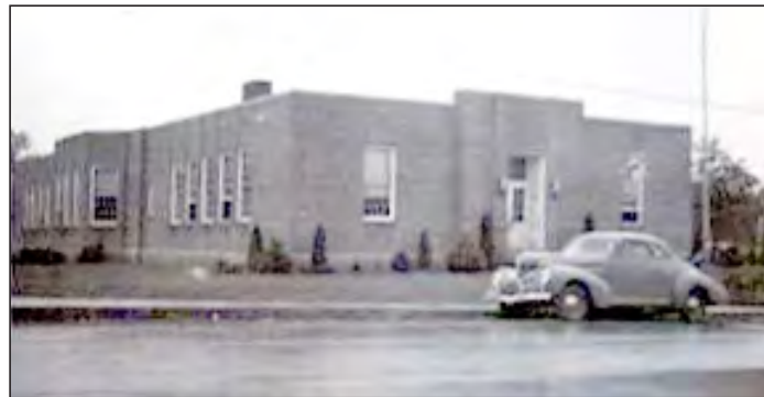
West Annapolis Elementary School, 1939 structure
